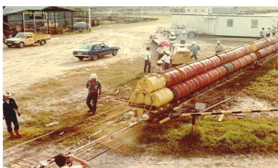
Launching of pipeline bundle from stringing yard 2 km from sea to the landfall
