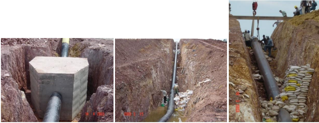
Installation of onshore section of pipeline and anchor block
