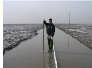
Pulling of pipeline with spoilers to landfall – notice that pipeline has self-buried due to spoilers
