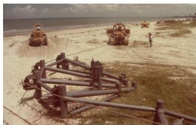
Launching of pipeline bundle from stringing yard 2 km from sea to the landfall
