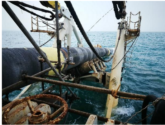
Typical pipelay activities (initiation, normal lay and preparation for laydown)
