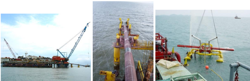
Laying of 28" pipeline and subsequent trenching by jetsled
