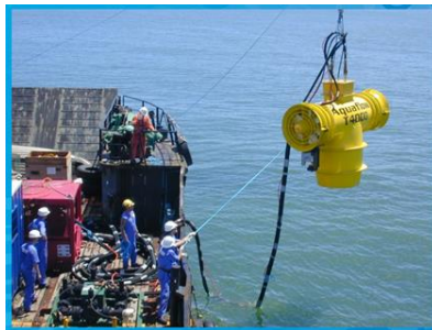
Jetting by Mass-flow Excavator of backfill cover on existing pipeline to facilitate cutting, lifting and above-water tie-in between new and existing pipeline segments
