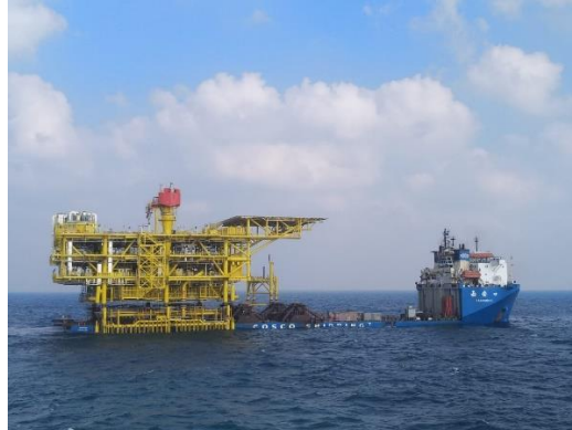
Platform installation by float-over method
