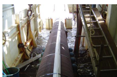
Installation of pipeline with spoilers
