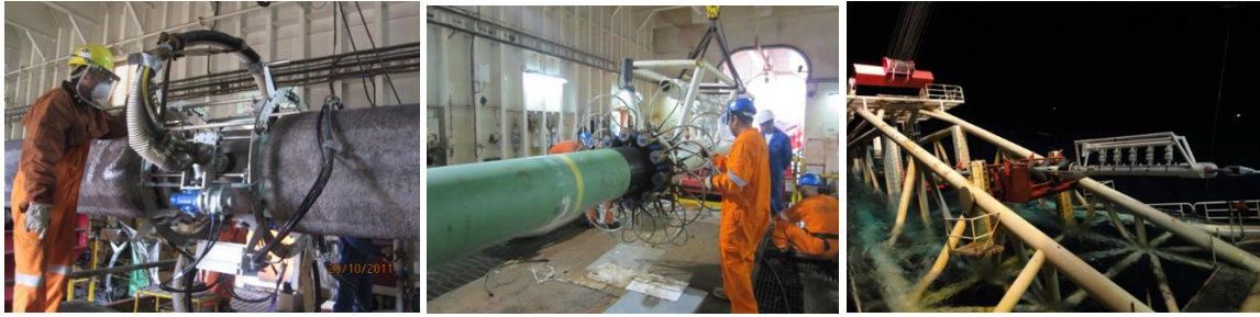
Pipeline installation (field joint coating, laydown head bolting & laydown of pipeline)
