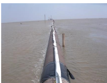
Pulling of pipeline with spoilers to landfall – notice that pipeline has self-buried due to spoilers
