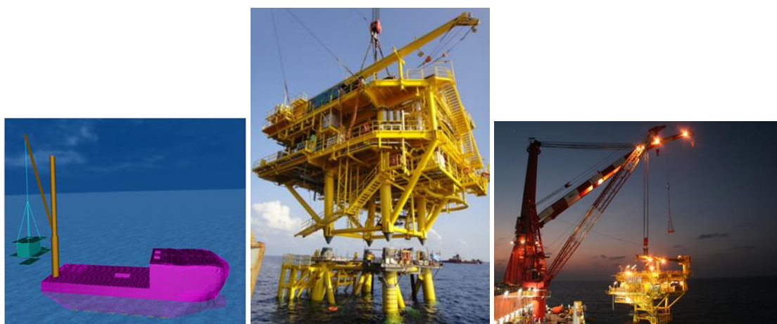
Engineered Lift Analysis using High-end Software and Actual Photos from Site
