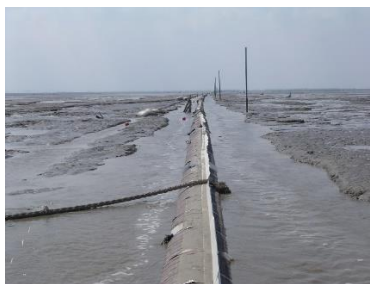
Pulling of pipeline with spoilers to landfall – notice that pipeline has self-buried due to spoilers
