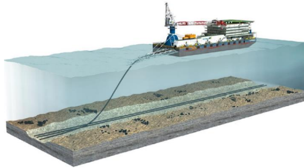
Laying of new 48" pipeline segment
