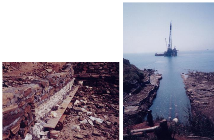
Approach to landfall was dredged and complex anchor mechanism made for multiple landings
