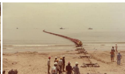
Launching of pipeline bundle from stringing yard 2 km from sea to the landfall
