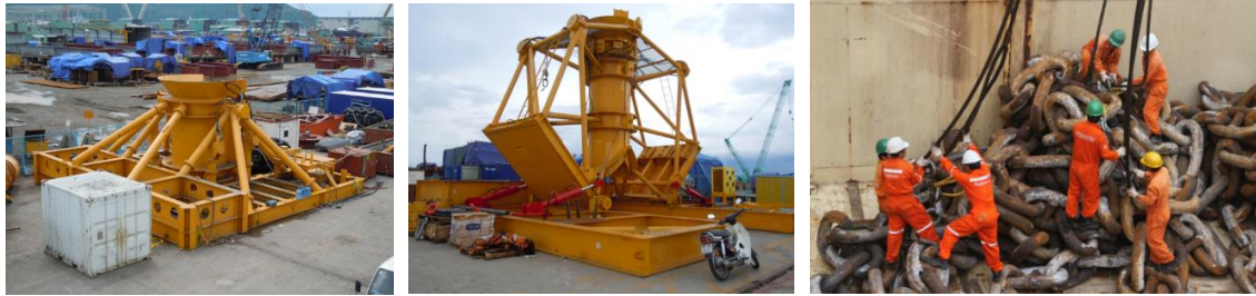
(Left & Middle) Pile handling frames for use offshore and (Right) Rigging chains inside vessel hold to offload the chains
