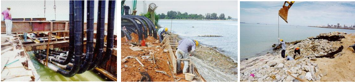
Riser Installation and Site Reinstatement after Completion of Bottom Pull
