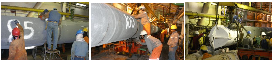
Welding addition pipe to recovered pipeline and preparation for abandonment
