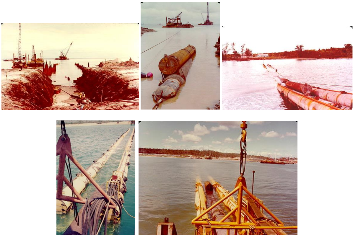
Examples of shore-pull for various pipelines installed during the campaign
