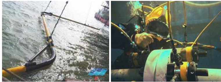
Installation of subsea spools
