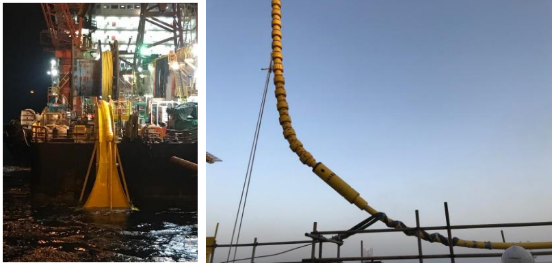
Installation of umbilicals
