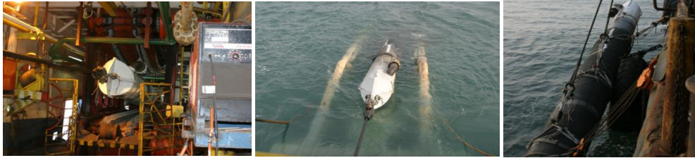
Abandonment of Pipeline & Subsequent Davit Lift for Tie-in to PLEM
