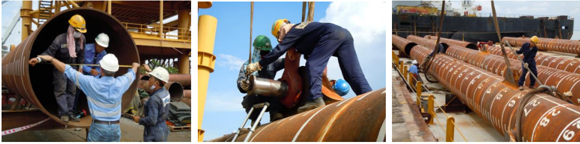
Confirmation of pile parameters before load-out onto material barge
