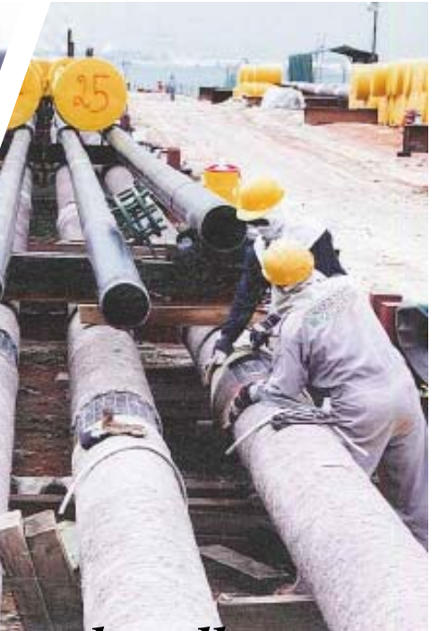
Alignment & tie-in of preceding bundle to the new bundle
