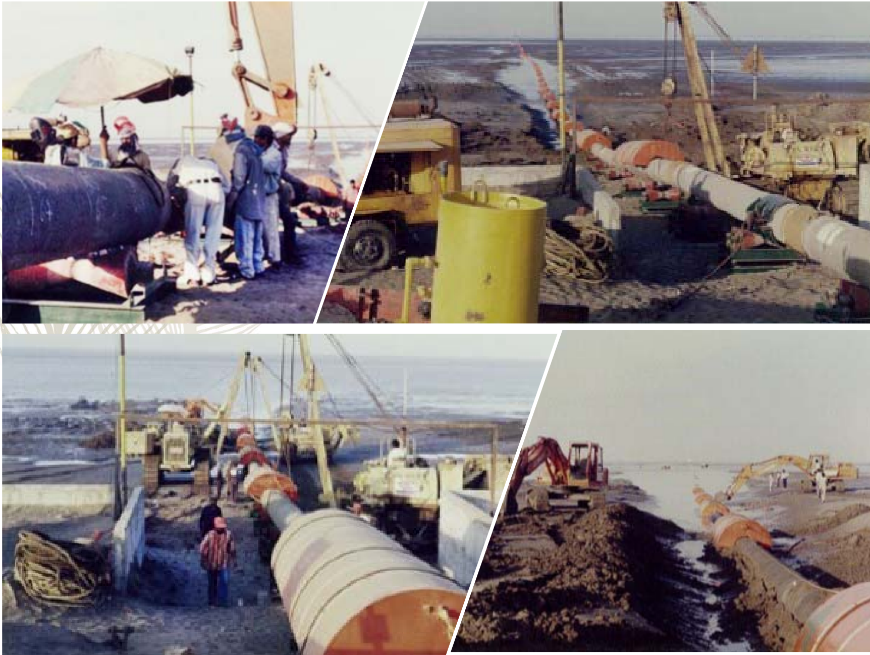
Welding of new pipe string to preceding string during low tide
