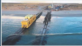
Controlled Depth Tow Method of Installation
