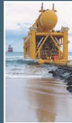
Surface-tow Method of Installation
