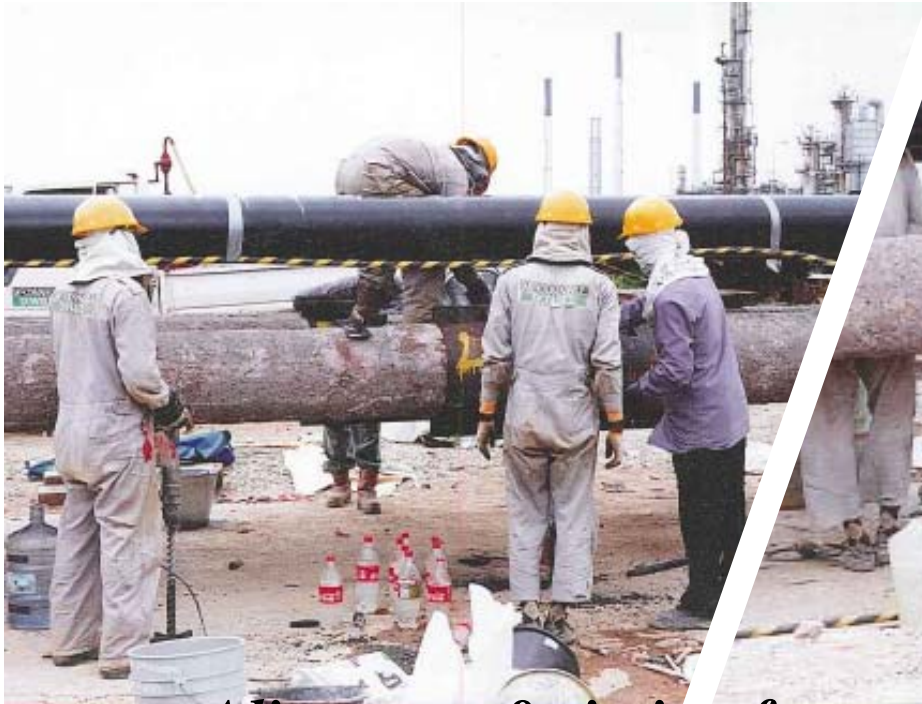
Alignment & tie-in of preceding bundle to the new bundle
