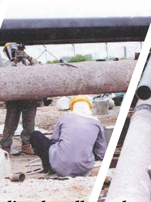
Alignment & tie-in of preceding bundle to the new bundle
