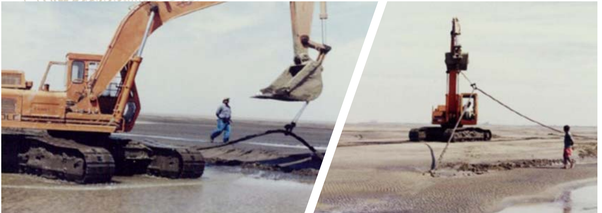
Dislodging pull cable from liquefiable soil & straightening it to reduce pull force
