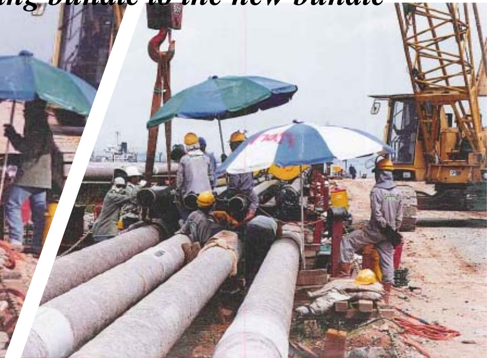
Alignment & tie-in of preceding bundle to the new bundle
