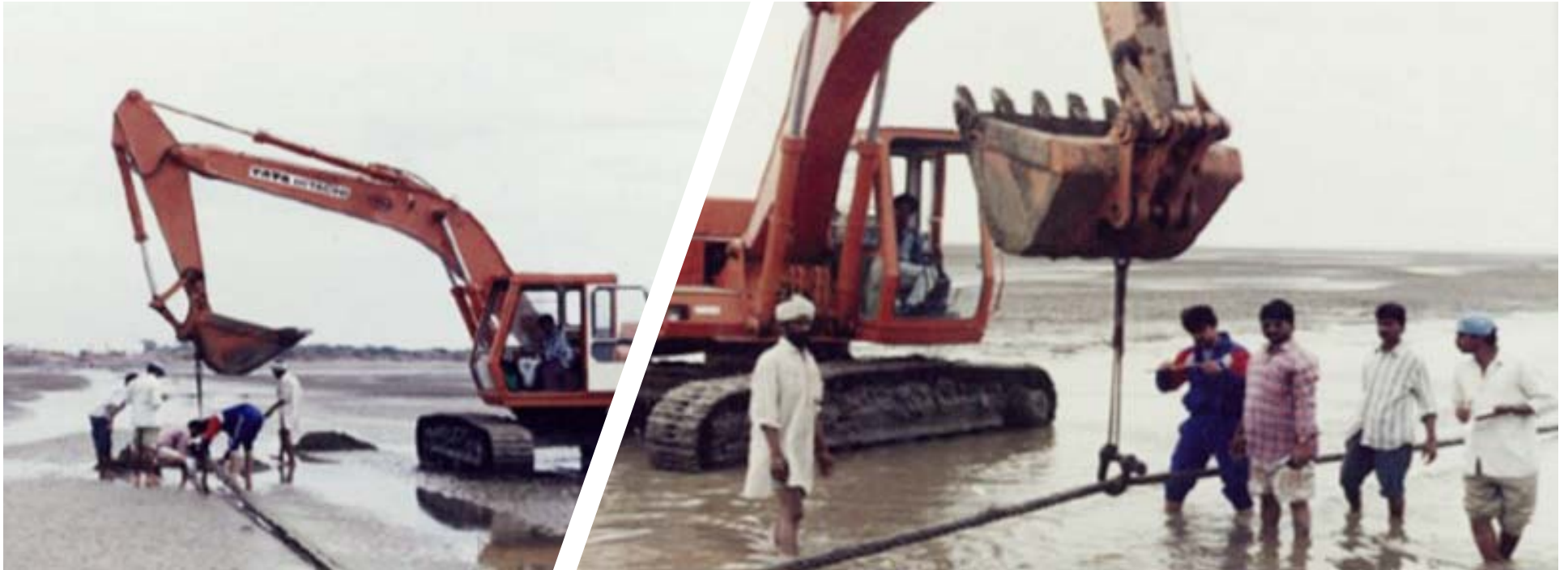
Dislodging pull cable from liquefiable soil & straightening it to reduce pull force
