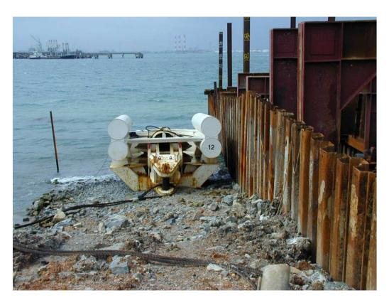
Sheave block enables effective pull force on pipe bundle to be double of the linear winch capacity
