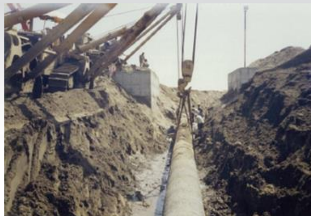
Lowering pipeline into trench
