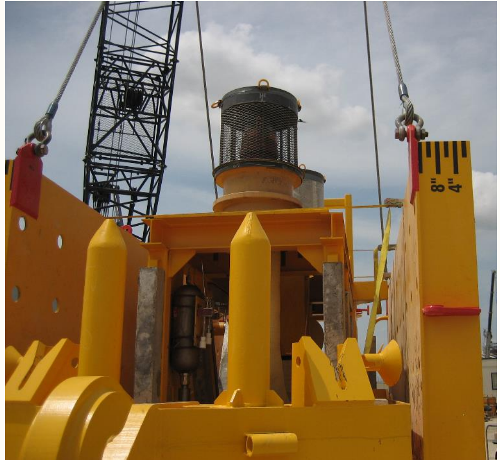
PLET Lift (Protective Cage Shown)
