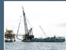
Stalk-on Method of Riser Installation
