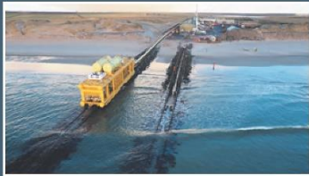
Controlled Depth Tow Method of Installation
