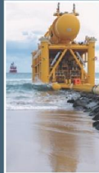
Surface-tow Method of Installation
