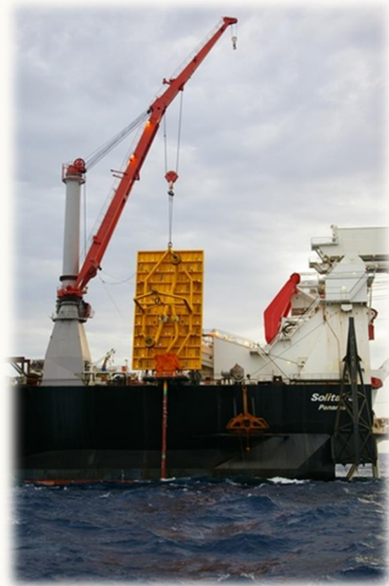
PLET Installed by J-mode
