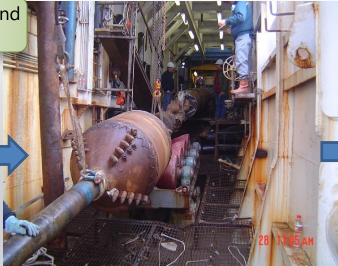
Swabber and pipeline pulled back to shore
