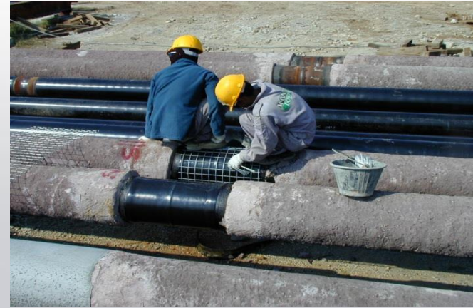
Pullhead for Pipe Bundle
