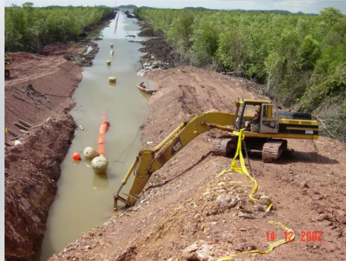
Completion of PUSH-PULL Installation & Reinstatement
