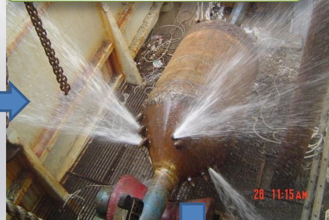
Swabber and pipeline pulled back to shore
