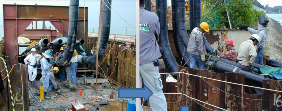
Installation of Risers on Pipe Bundle
