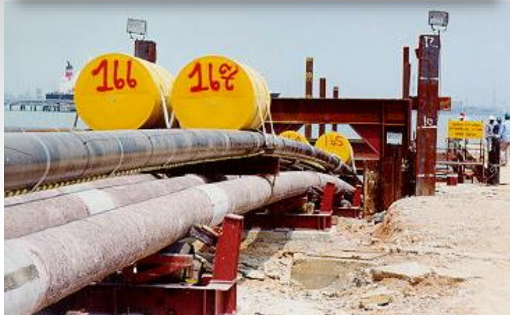
Pipe Bundle (with BT) on Launch way
