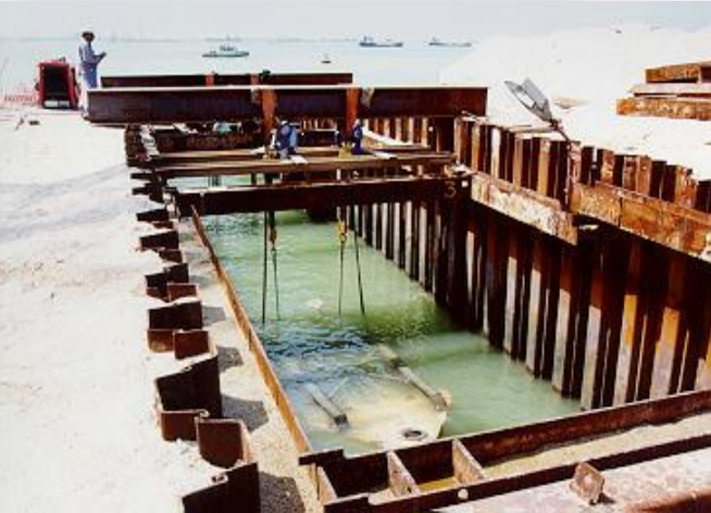
Arrival of Pulling Head
