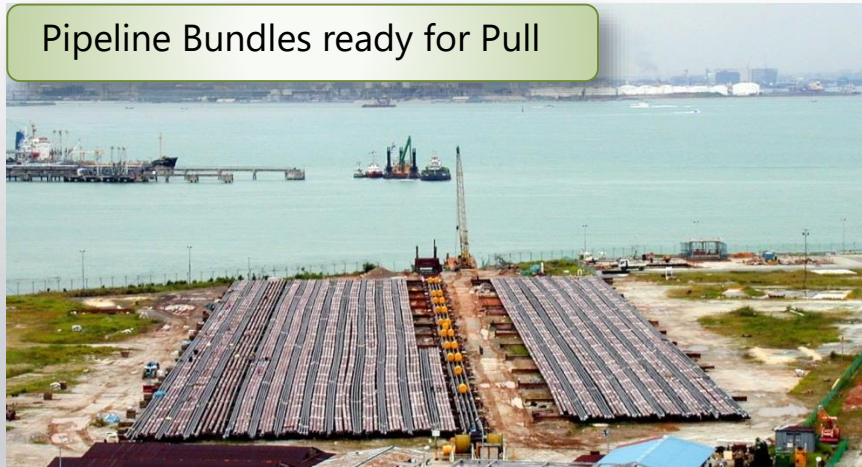
Pipe Bundle (with BT) on Launch way
