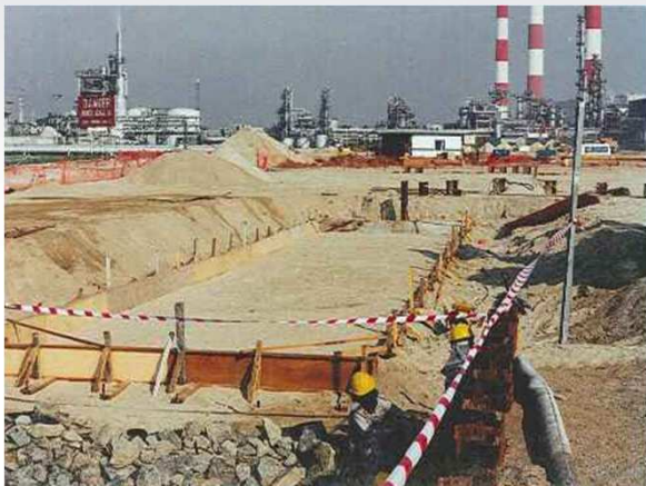
Linear Winch Base Construction and Arrangement for Pipe Pull
