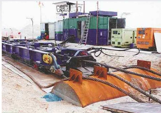
Linear Winch Base Construction and Arrangement for Pipe Pull
