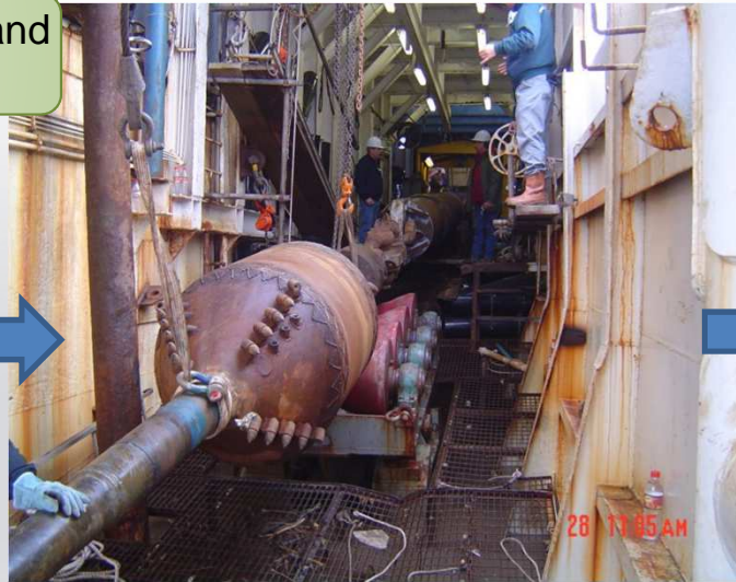
Swabber and pipeline pulled back to shore
