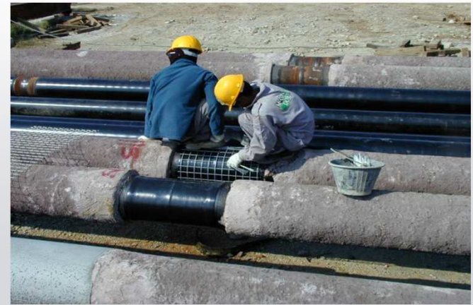
Pullhead for Pipe Bundle
