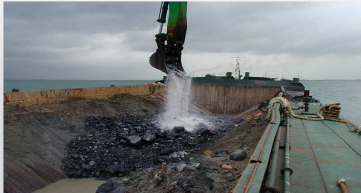
Drilling and Blasting Works along Pipeline Route to shatter rocks to enable Dredging
