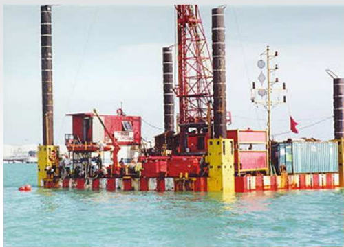
Drilling and Blasting Works along Pipeline Route to shatter rocks to enable Dredging
