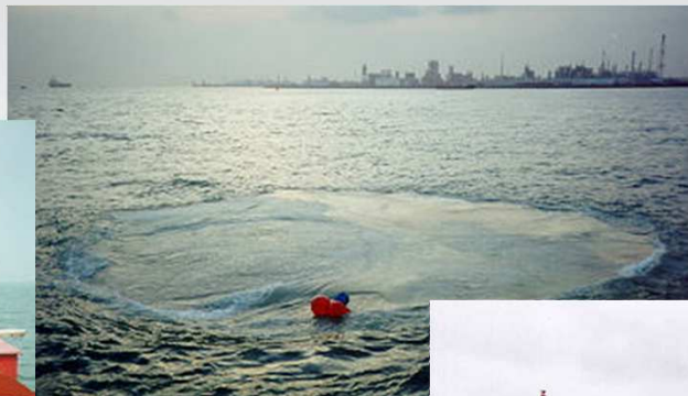
Drilling and Blasting Works along Pipeline Route to shatter rocks to enable Dredging
