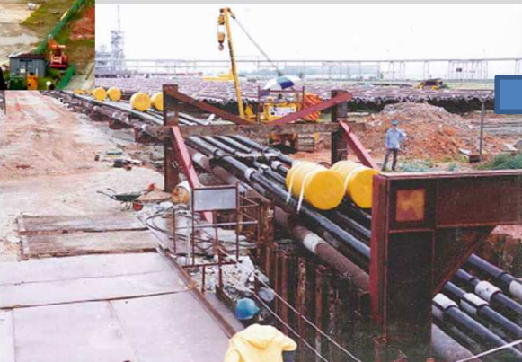
Pipe Bundle (with BT) on Launch way
