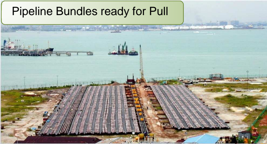
Pipe Bundle (with BT) on Launch way
