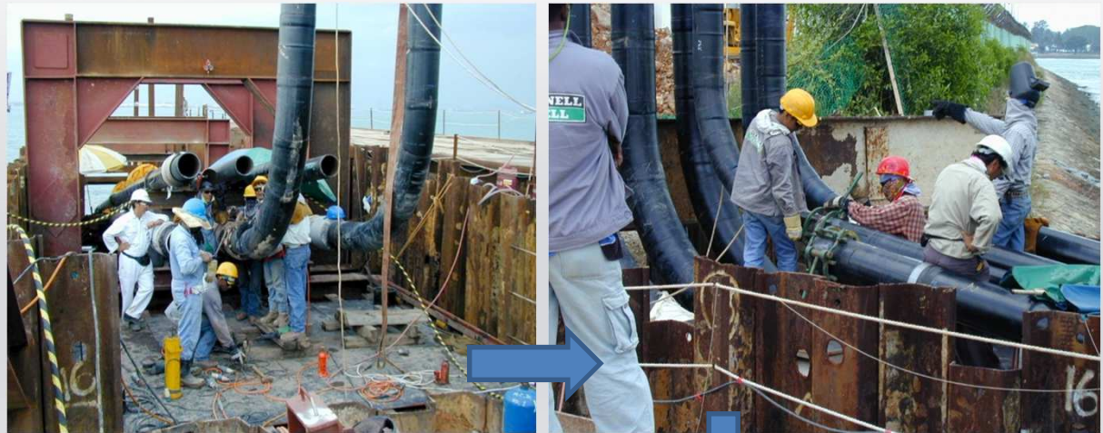
Installation of Risers on Pipe Bundle
