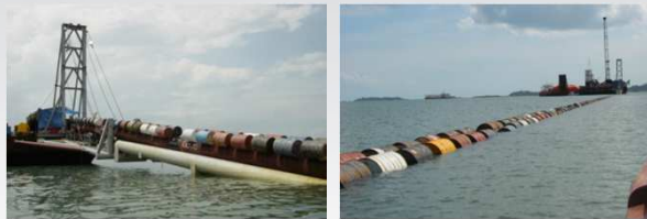
Buoyancy Drums to Provide Positive Buoyancy
