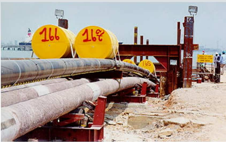
Pipe Bundle (with BT) on Launch way
