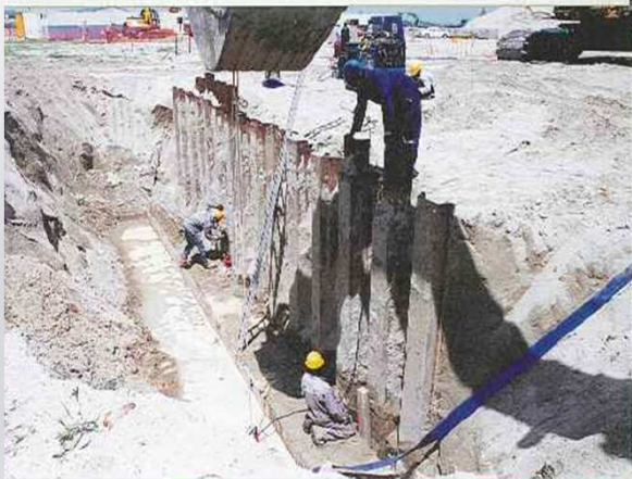
Linear Winch Base Construction and Arrangement for Pipe Pull
