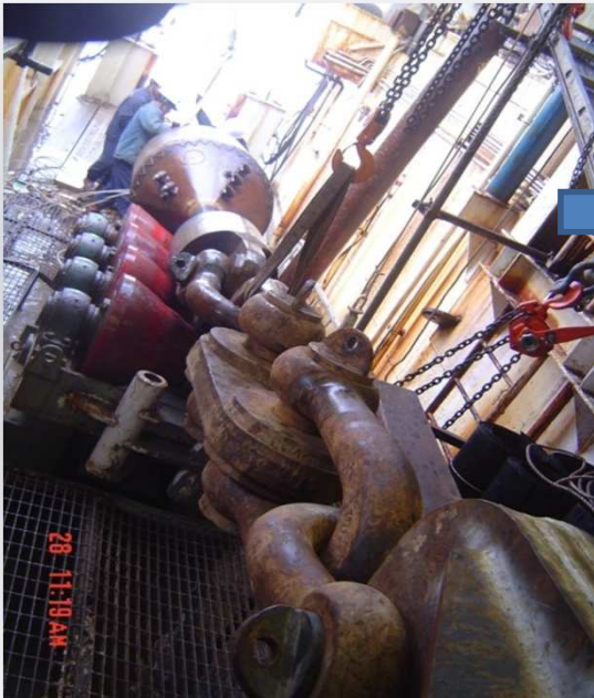
Swabber/ reamer on laybarge and connected to pullhead
