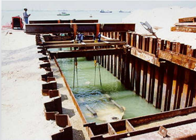
Arrival of Pulling Head
