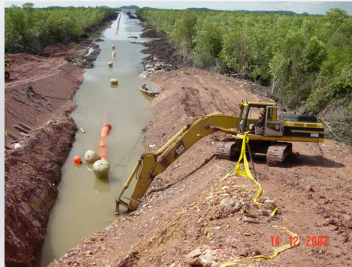
Completion of PUSH-PULL Installation & Reinstatement
