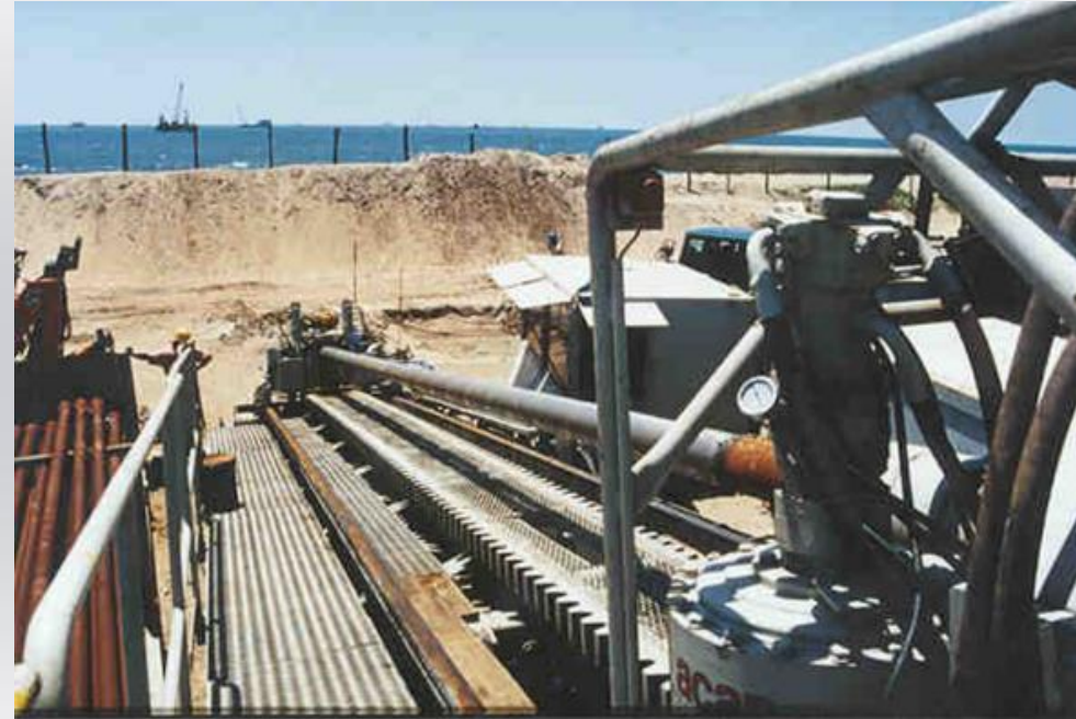
An example of landfall HDD operation for installing pipeline at shore approach
