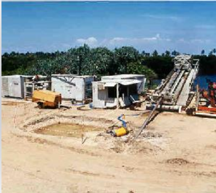
An example of landfall HDD operation for installing pipeline at shore approach
