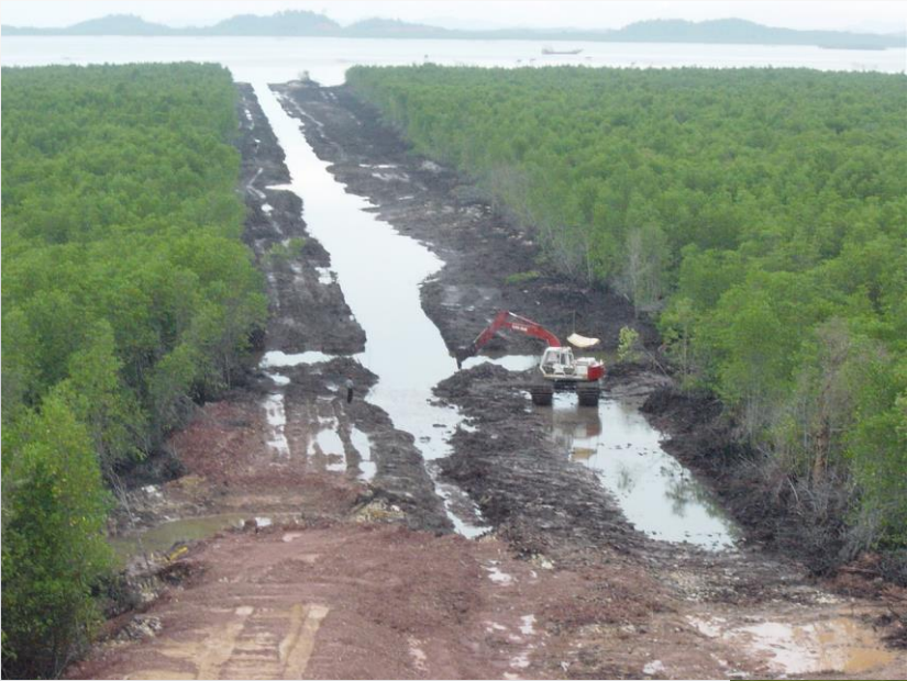
Backfilling after Pipeline has been Installed
