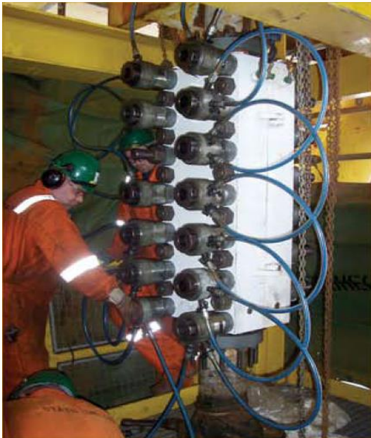
Typical Dual Seal Repair Clamp from STATS Group
