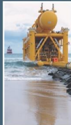
Surface-tow Method of Installation
