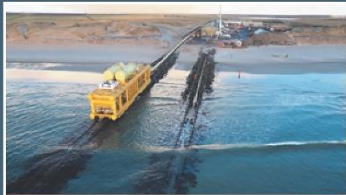
Controlled Depth Tow Method of Installation
