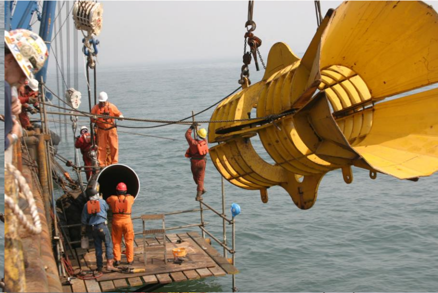
Preparing pipe end for riser add-on; stabbing guide attach to assist with riser spool/riser bend alignment & subsequent welding
