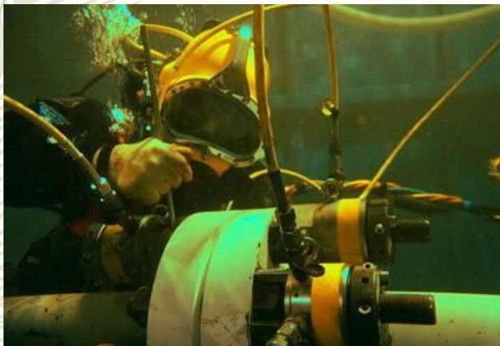
Underwater bolt tightening using Hydratight bolt tensioning equipment.
