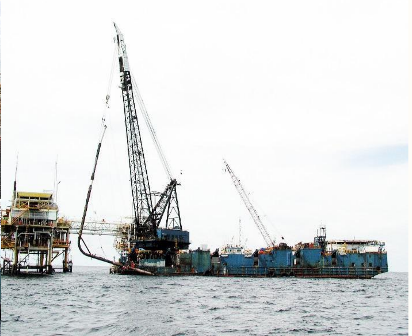
Lifting of riser assembly and stalking-on to pipe end for welding
