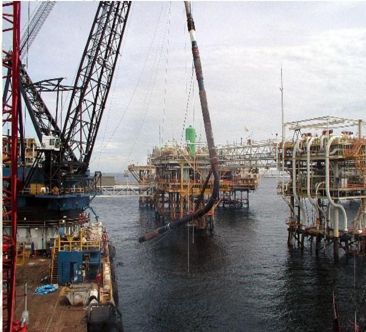
Lifting of riser assembly and stalking-on to pipe end for welding
