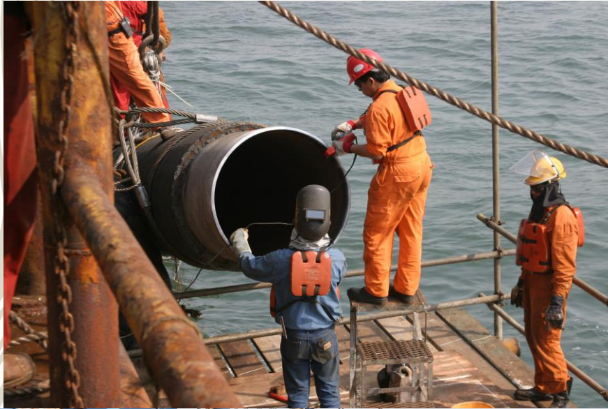
Preparing pipe end for riser add-on; stabbing guide attach to assist with riser spool/riser bend alignment & subsequent welding
