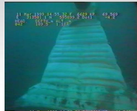
Typical Grout Bags for Span Corrections
