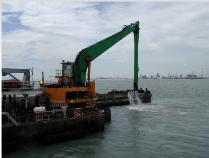
Van Oord's Backhoe Dredger "Ave Caesar" dredging rocky seabed in Singapore & 2 no. hopper barges for disposal of spoils
