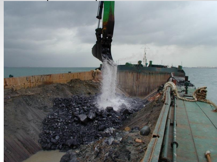
Van Oord's Backhoe Dredger "Ave Caesar" dredging rocky seabed in Singapore & 2 no. hopper barges for disposal of spoils
