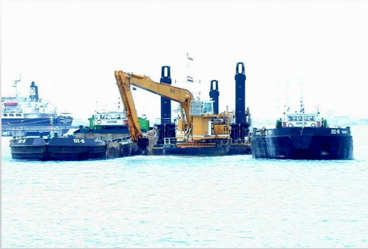
Van Oord's Backhoe Dredger "Ave Caesar" dredging rocky seabed in Singapore & 2 no. hopper barges for disposal of spoils
