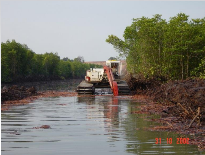
Shore approach / mangrove swamp dredging using 'march buggy'
