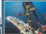
S-lay Method of Installation
