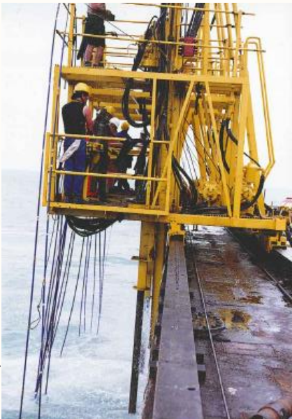
Note cables hanging from drilling m/cs to sea. Those are detonation control cables to initiate the detonation.
