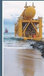
Surface-tow Method of Installation
