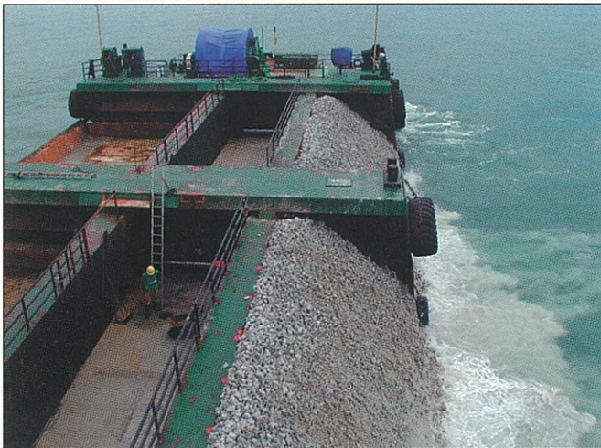
Filterlayer vessel (above, left) dumps rock over the laid pipeline bundle (Fig. 5). Backhoe dredger (above, right) works in advance of pipelay operations (Fig. 6). Photographs from Kvaerner E&C, Singapore.
