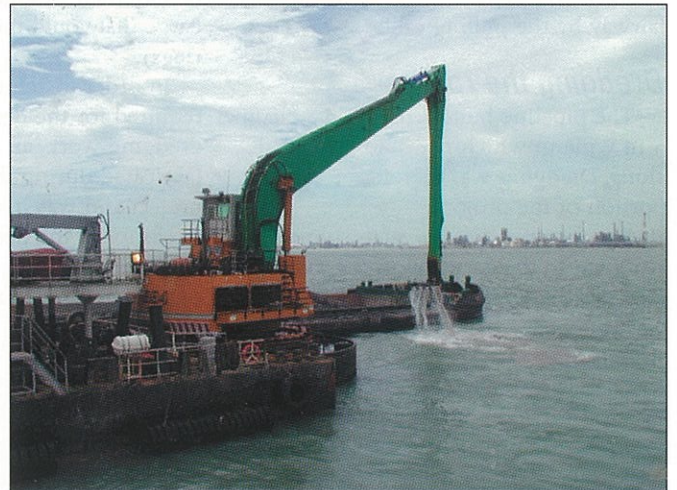
Filterlayer vessel (above, left) dumps rock over the laid pipeline bundle (Fig. 5). Backhoe dredger (above, right) works in advance of pipelay operations (Fig. 6). Photographs from Kvaerner E&C, Singapore.
