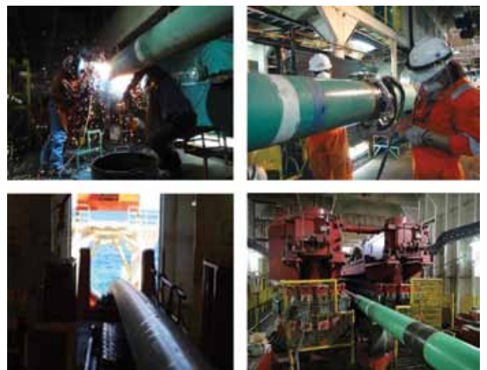
Figure 4: S-Lay Typical Process (Clockwise from Top Left): (a) Welding; (b) Welding Inspection/ Test; (c) Going through Tensioner; (d) Pipeline Going through Stinger before Lift-Off
