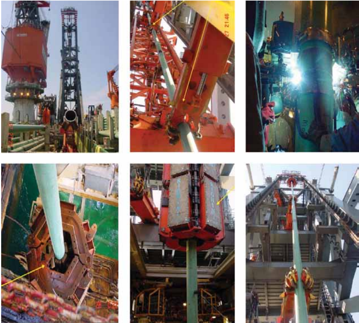
Figure 8: J-Lay Typical Process (Clockwise from Top Left): (a) Upending of Pre-Assembled Quad Joints (b) Line-Up in the J-Lay Tower and Clamped; (c) Welding (and NDT) in Vertical Position; (d) Preparation of Next Proceeding String; (e) Snapshot of Travelling Clamp; (f) Going through Hang-Off Clamp.
